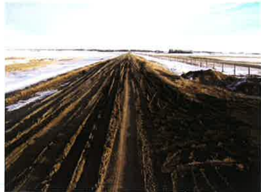
Fig. 5 County of Wetaskiwin Road damage from oil and gas drilling
